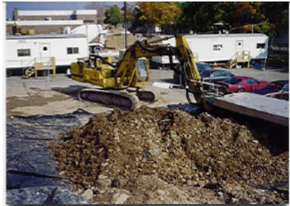
Above Ground Soil Mixing MITU 12
