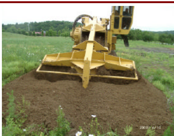
In-Place Soil Mixing MITU-LVR
