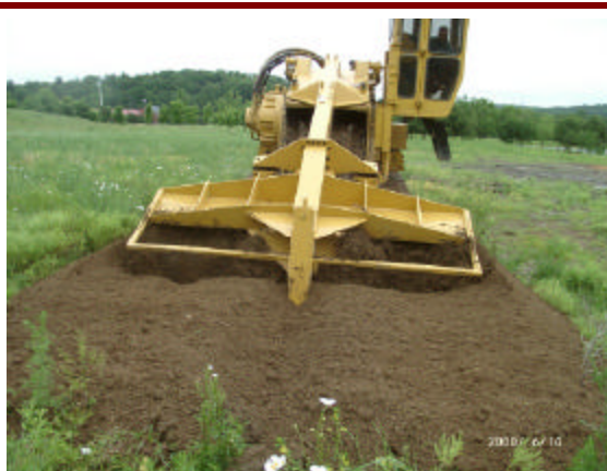
In-Place Soil Mixing MITU-LVR
