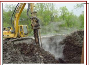
MITU-12 mixing KMnO<sub>4</sub> with CVOC contaminated soil in Milwaukee, WI
