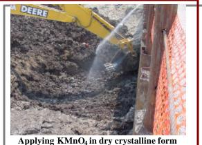
Applying KMnO4 in dry crystalline form Milwaukee, WI
