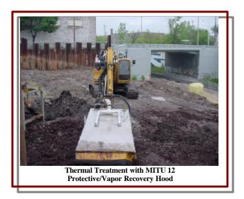
Typically, there is no combustion involved in either the primary or secondary treatment of organics with the MITU; therefore, air quality permitting is of minor significance. However, for contaminants with low adsorption isotherms, secondary catalytic or thermal oxidation of the vapor stream may be required. If necessary, CBA has experience in obtaining the proper air quality permits for utilization of the MITU.
